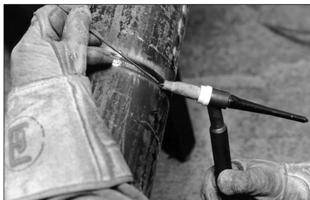
Figure 8.13 Demonstration of how the torch and filler rod are held to accomplish the “walking-the-cup” method of pipe welding.
