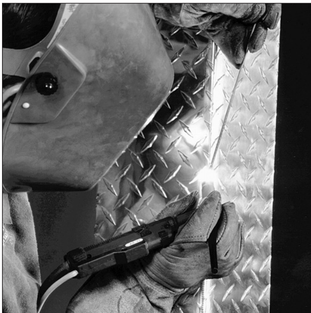
Figure 8.9 Welding in the vertical position.
