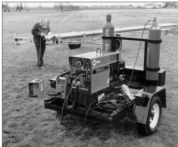
Figure 3.16 Maintenance welding on agricultural equipment with an engine driven power source.
