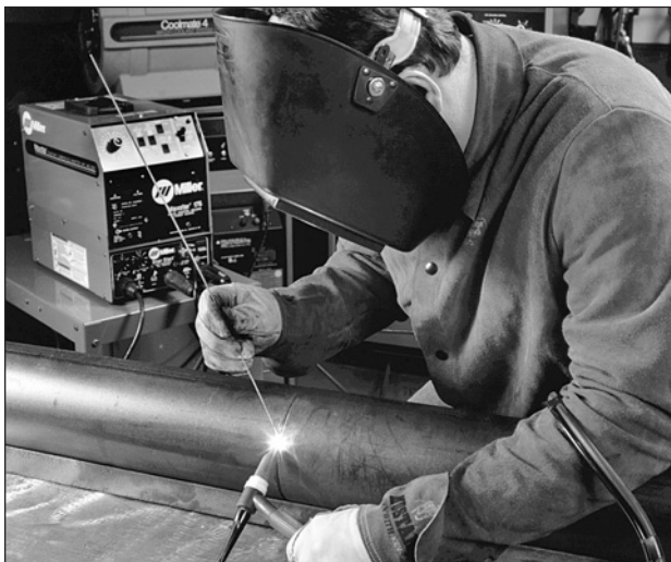
Figure 8.14 This welder (who happens to be left handed) demonstrates still another style of torch and filler rod manipulation used to accomplish a pipe weld.
